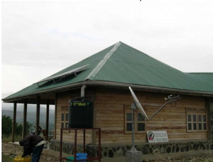
PV array, rainwater catchment, VSAT dish
